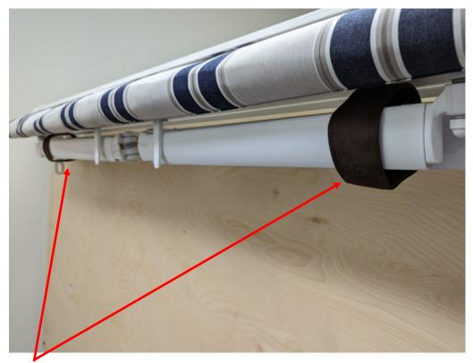
**Step 3**—Using tape or other material, retain the arms so that they can not spring out when motor is removed. Turn the manual override to let the awning fabric and arms out to remove tension from the motor.
