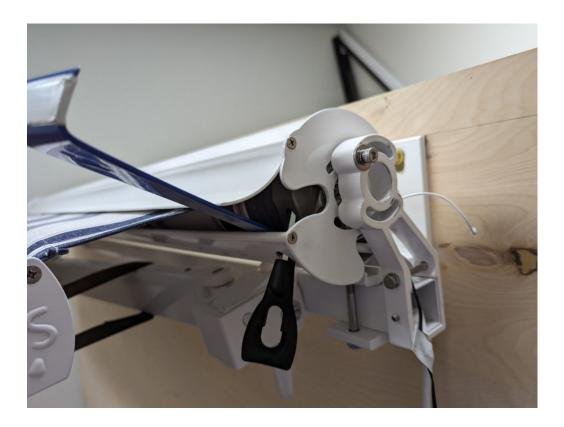
**Step 11**—Slide awning end bracket back on mounting tube. Using a prybar, gently li the roll tube and housing upwards into place and start the round allen screws into the bracket.
